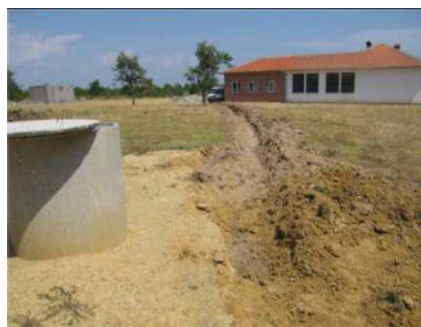
The well, trench and school
